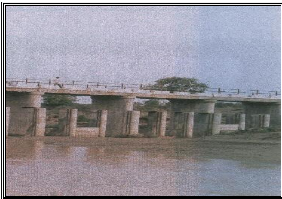
Typical arrangement of Bandhara piers
