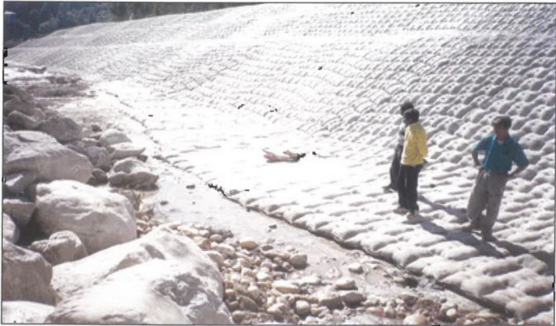
Figure A12. Photograph of Fabric Form Mattress with Launching Apron on River Bed
