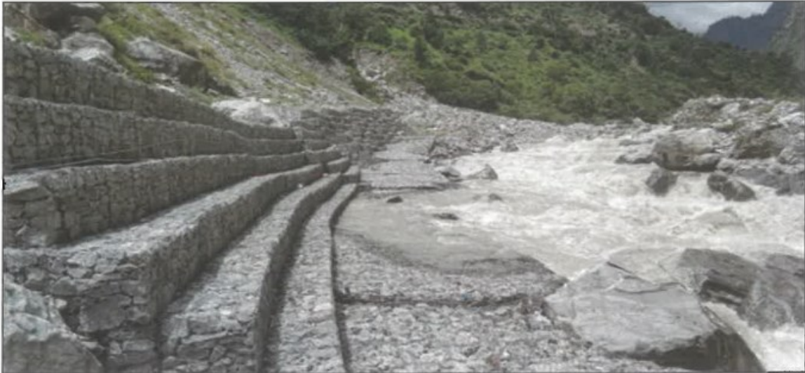
Figure A10. Photograph of Gabion Retaining Wall with Launching Apron on River Bed
