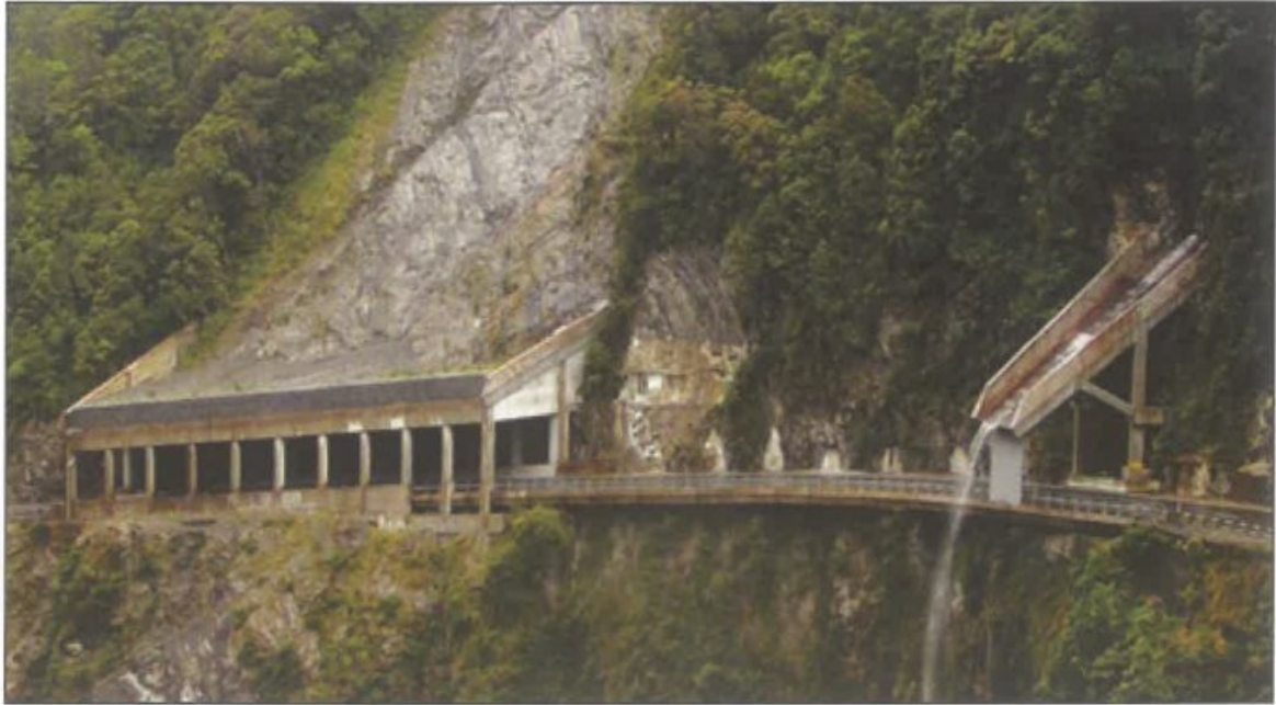
Figure A4. Site Photograph of Rock Shed
